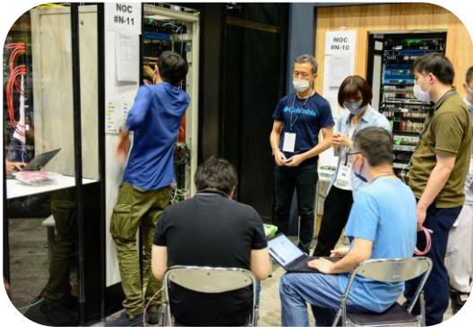
Setup and construction of equipment
