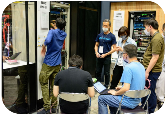
Setup and construction of equipment
