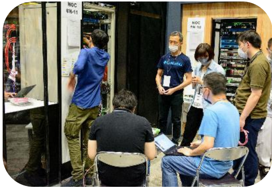
Setup and construction of equipment
