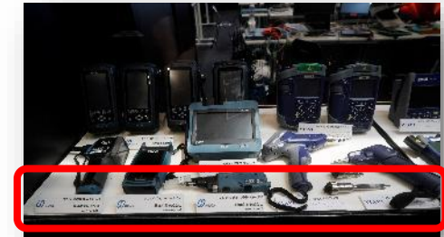
Non-rack mounted equipment
